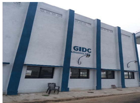
Water Supply facility in Bhagapura, funded by GIPP.
