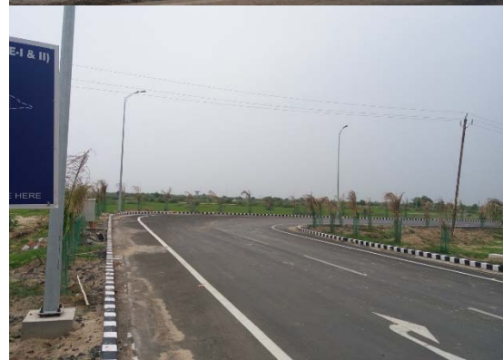
Khoraj Estate Road funded by GIPP
