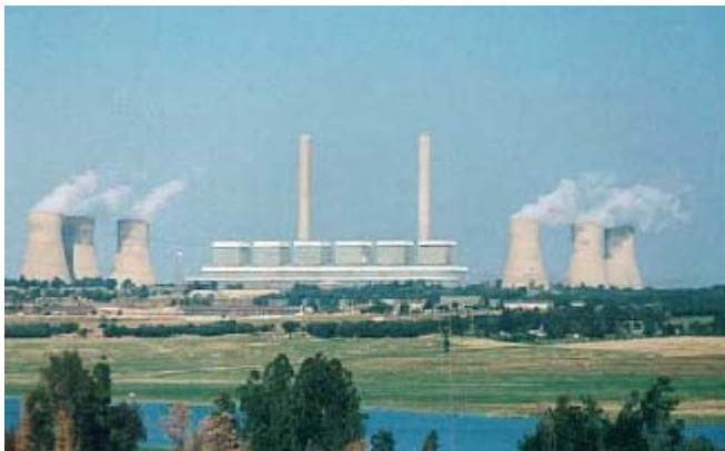
< South Africa CFB Power Station >
